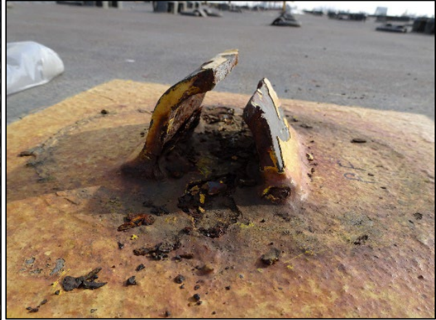
Figure 4. Failed Securing Strap
